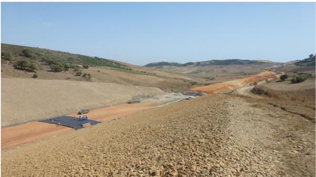
5. Global view of the work site : Great Speed Line Tanger - Kenitra
