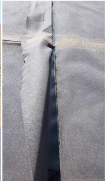
4. Over lapping of the PROTECTERRE PG
