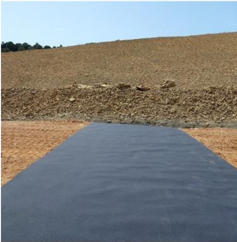
3. Laying of PROTECTERRE PF on the work site.
